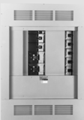
I-Line® Panelboards Page 9-20
